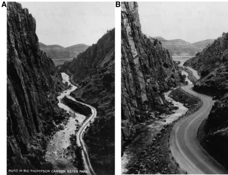
Figures 5a and 5b. The Big Thompson Canyon route ca. 1910 (left) and ca. 1940 (right) at the gorge's mouth. Note the channel constriction of the Big Thompson River due to the massive amounts of earth moved to construct US Highway 34. Credit: Fort Collins Museum of Discovery Archives.
