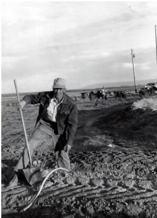
Fig. 6: Joe Flood takes a moment to rest while digging a ditch, 1954.
