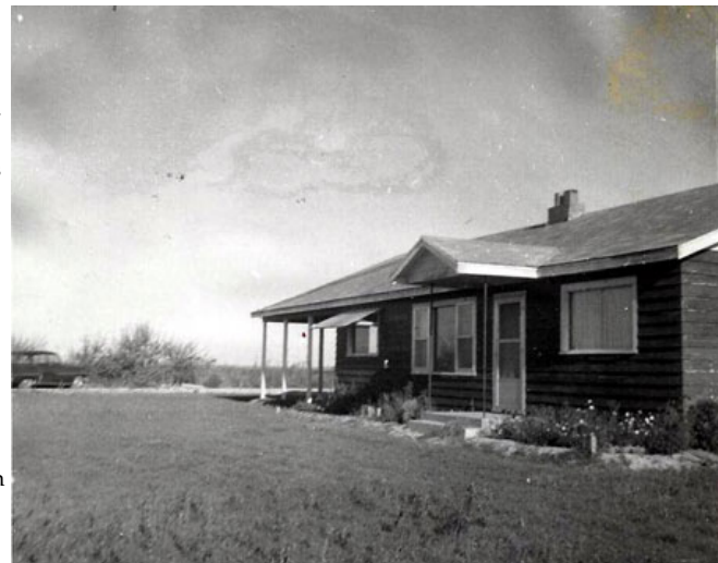
Fig. 10: The Flood's house, shortly after it was completed, 1955. Courtesy of Barbara Adams, Rupert, Idaho.
